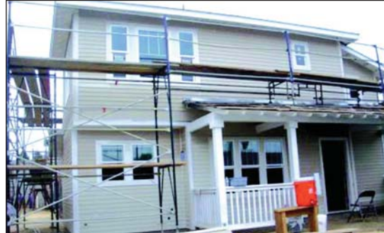
One of four condos being built on Sherman Ave. in Monrovia.
